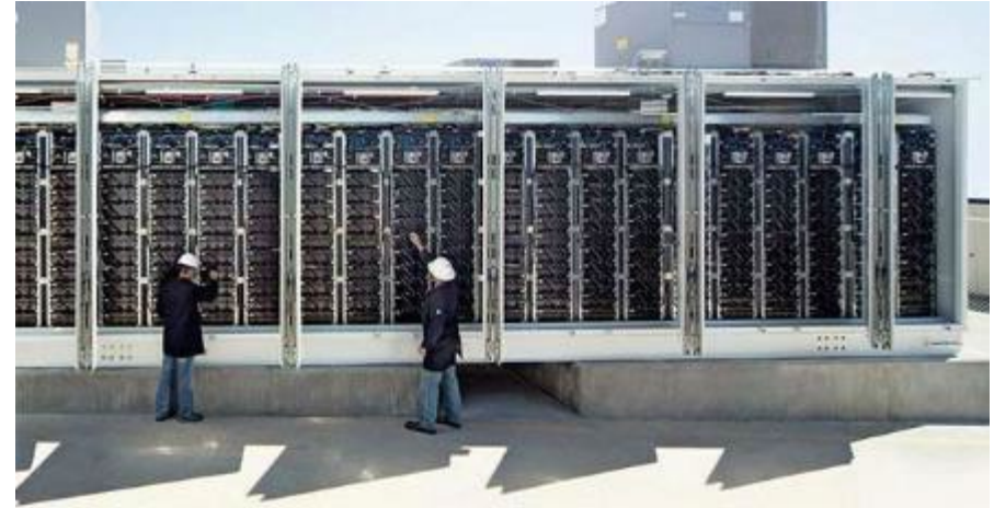
Example Lithium-Ion Battery Racks
