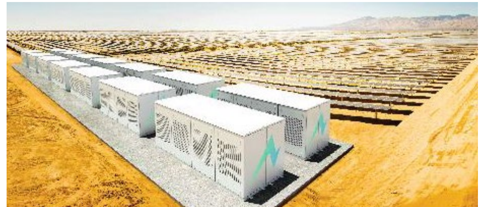
Example BESS + PV Project Site
